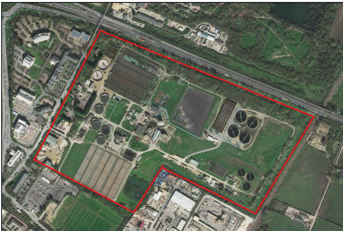
Figure 2.1 Existing WWTP site
